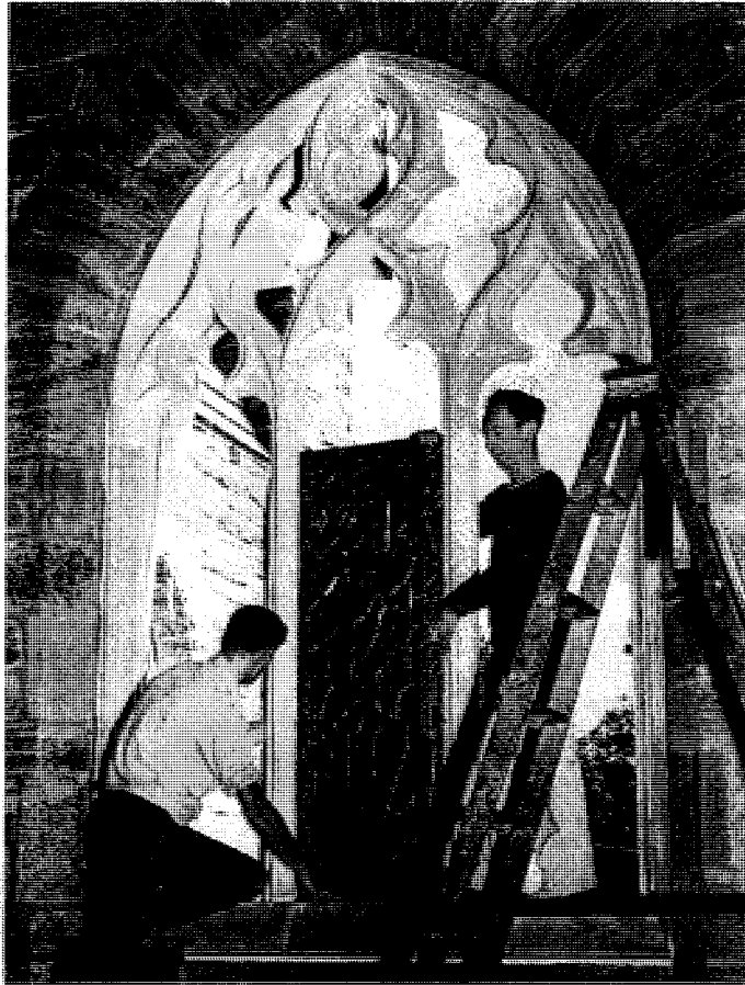
Installing A Stained Glass Window
