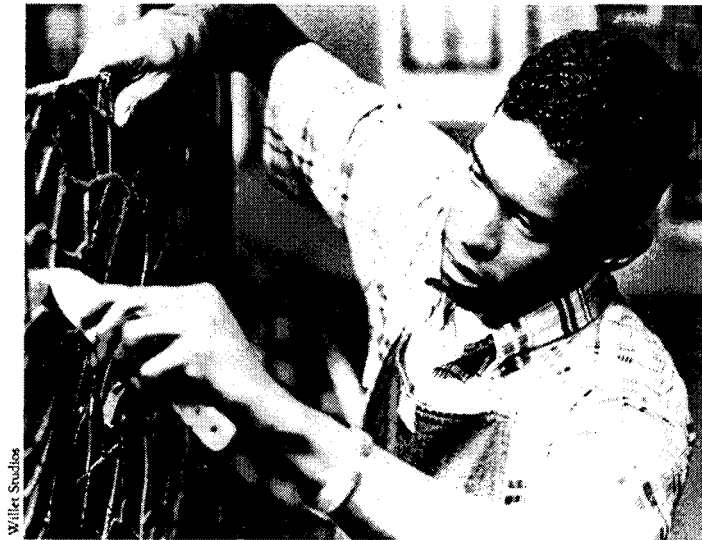
Cleaning a section of leaded stained glass that has just been puttied.
