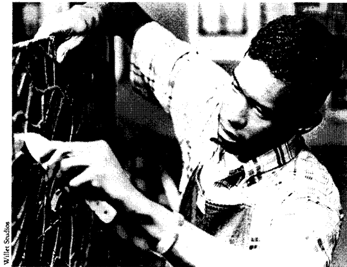
Cleaning a section of leaded stained glass that has just been puttied.
