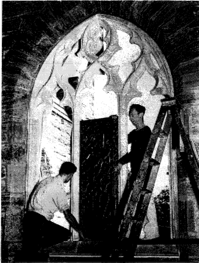
Installing A Stained Glass Window
