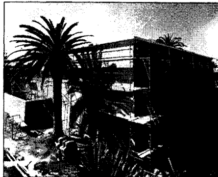
Construction of new Museum.
