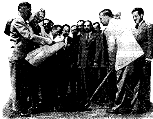
The Groundbreaking: On August 20, 1948, Emperor Ralph M. Lewis turned the first shovelful of soil on the site of the new temple, while other officers of the Supreme and Grand Lodges witnessed the event.
