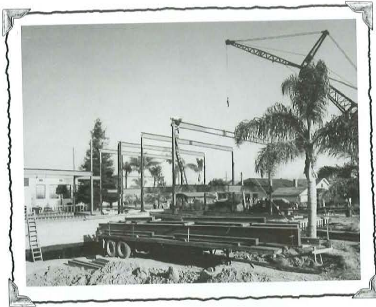
Much-enlarged Rosicrucian Egyptian Museum under construction in 1966.
