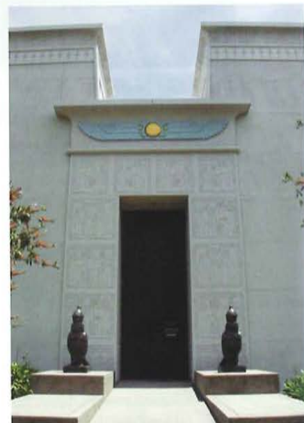
AMORC Administration Building: The "Institution Behind the Organization." Exterior repainted 2004. Funded by the Campaign for Rosicrucian Park.
