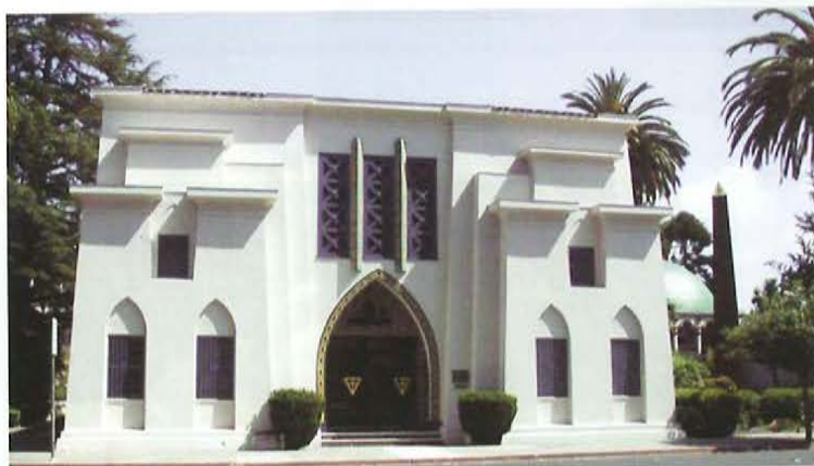
Francis Bacon Auditorium: Constructed in 1931, the auditorium's exterior was repainted in 2004. Funded by the Campaign for Rosicrucian Park.
